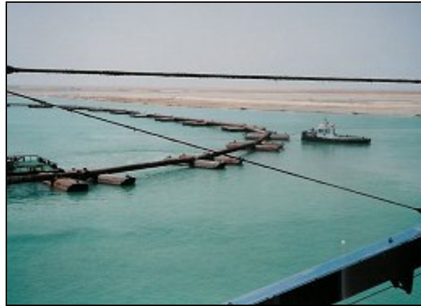
Fig. 4.2. Floating Pipelines used to Transport Dredged Materials from a CSD
